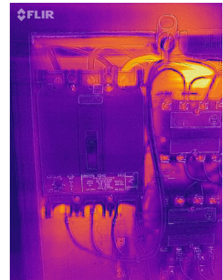
Identify electrical faults
